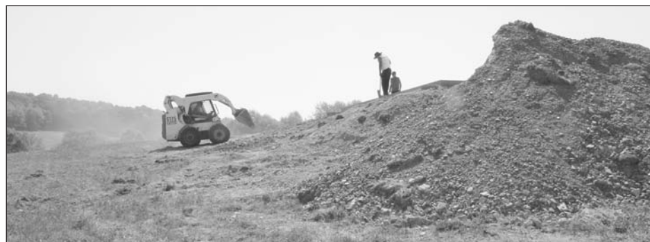
Workers fill around Our Lady of Mercy Church, under construction.
