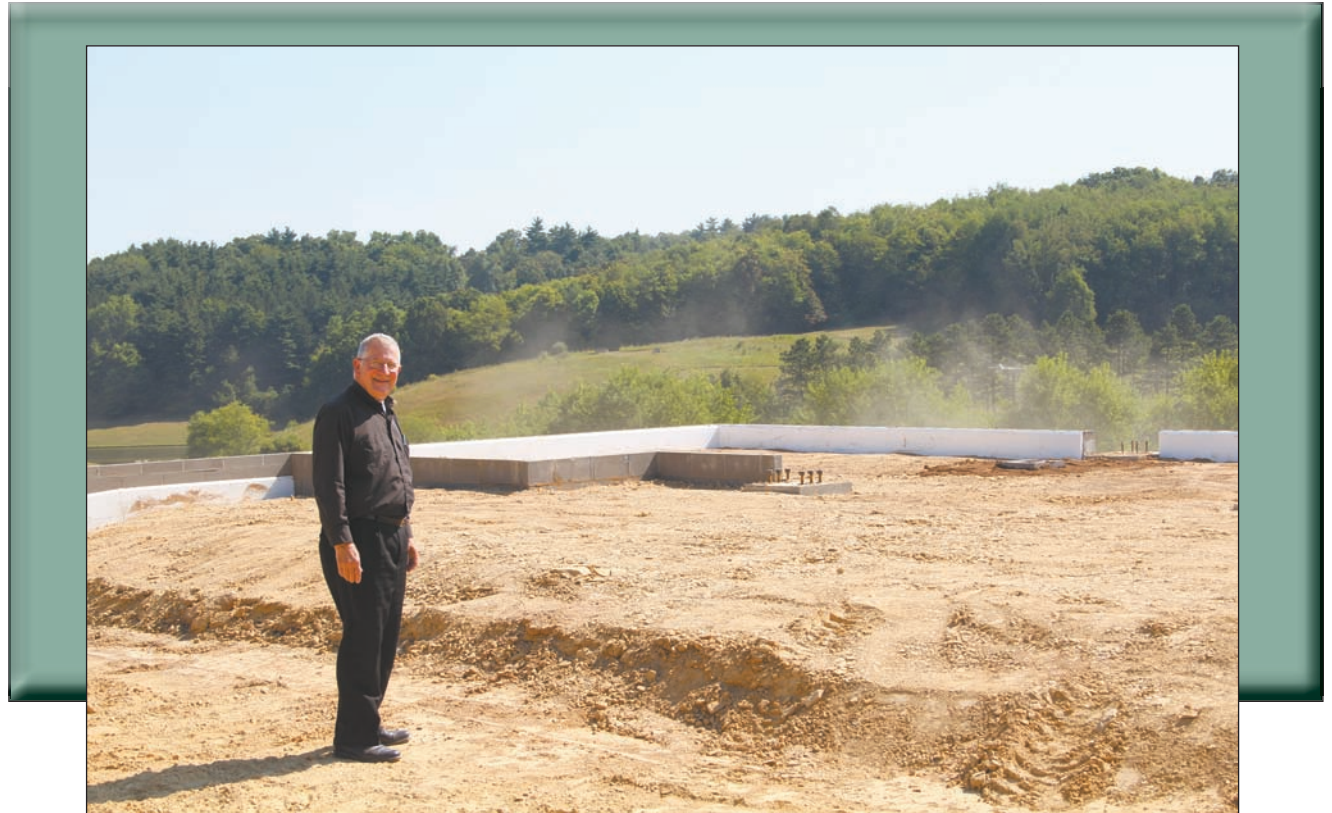
Father Anthony R. Batt, pastor of Our Lady of Mercy Parish, Carrollton, and St. Mary of the Immaculate Conception Parish, Morges, stands in front of where the altar will sit in the new Our Lady of Mercy Church, under construction in Carroll County. (Photo by DeFrancis)
