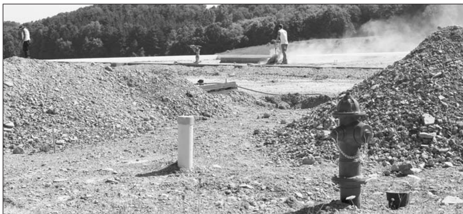
The foundation of Our Lady of Mercy Church is being shaped. (Photos by DeFrancis)
