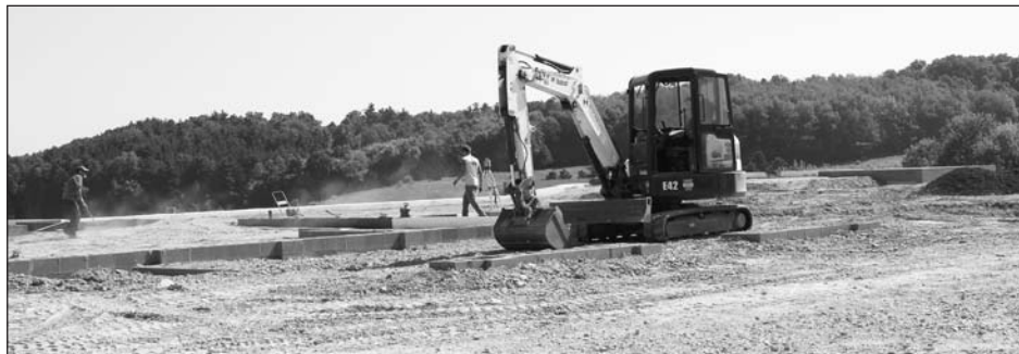
A piece of heavy equipment sits at what will be the entrance to Our Lady of Mercy Church.
